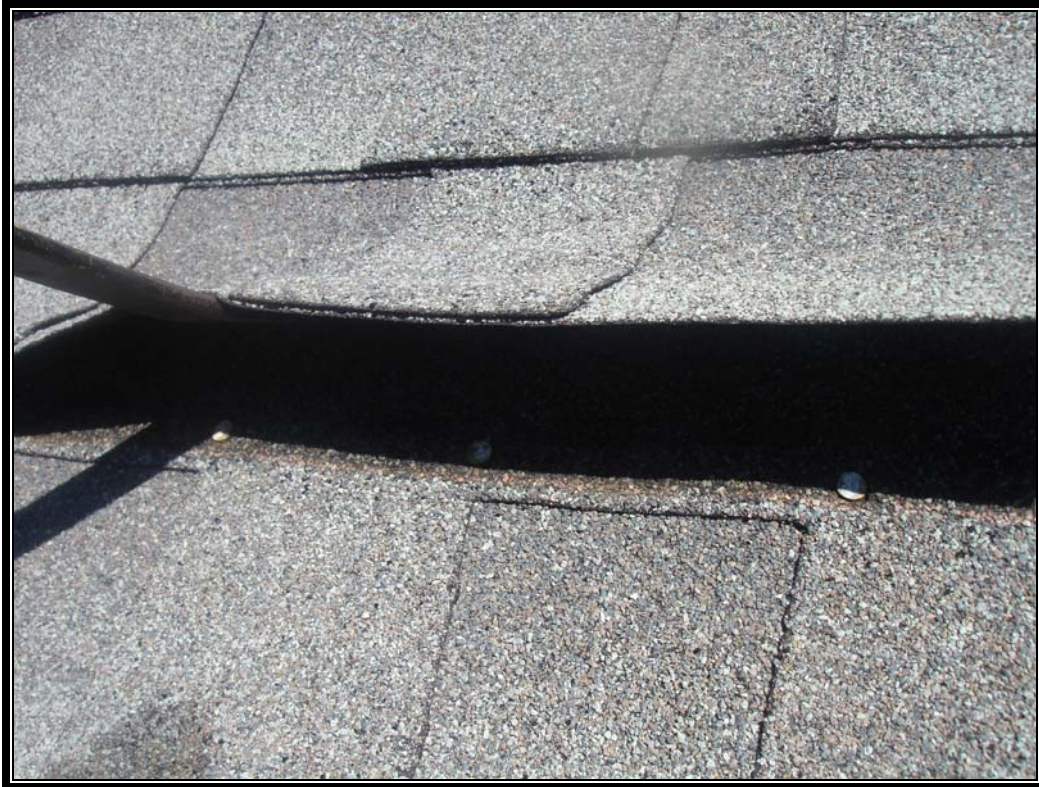
PHOTO #5: PROPER FASTENING PATTERN - TYPICAL
