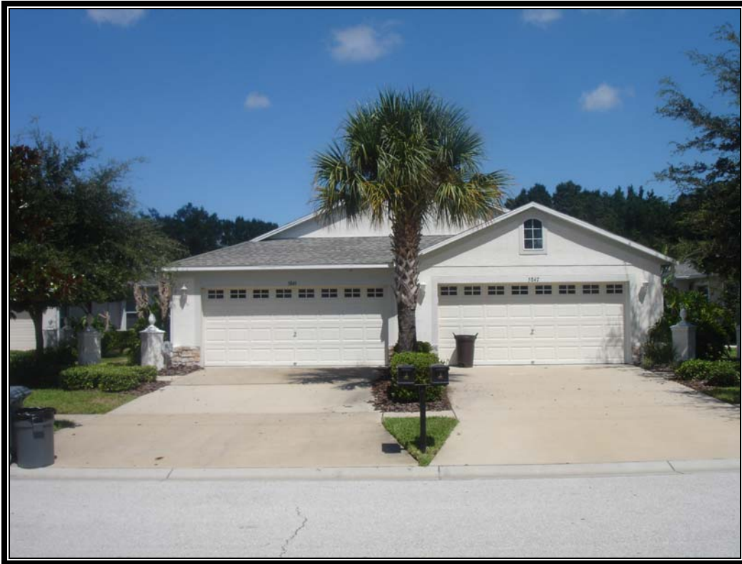
PHOTO #1: FRONT VIEW - TYPICAL
