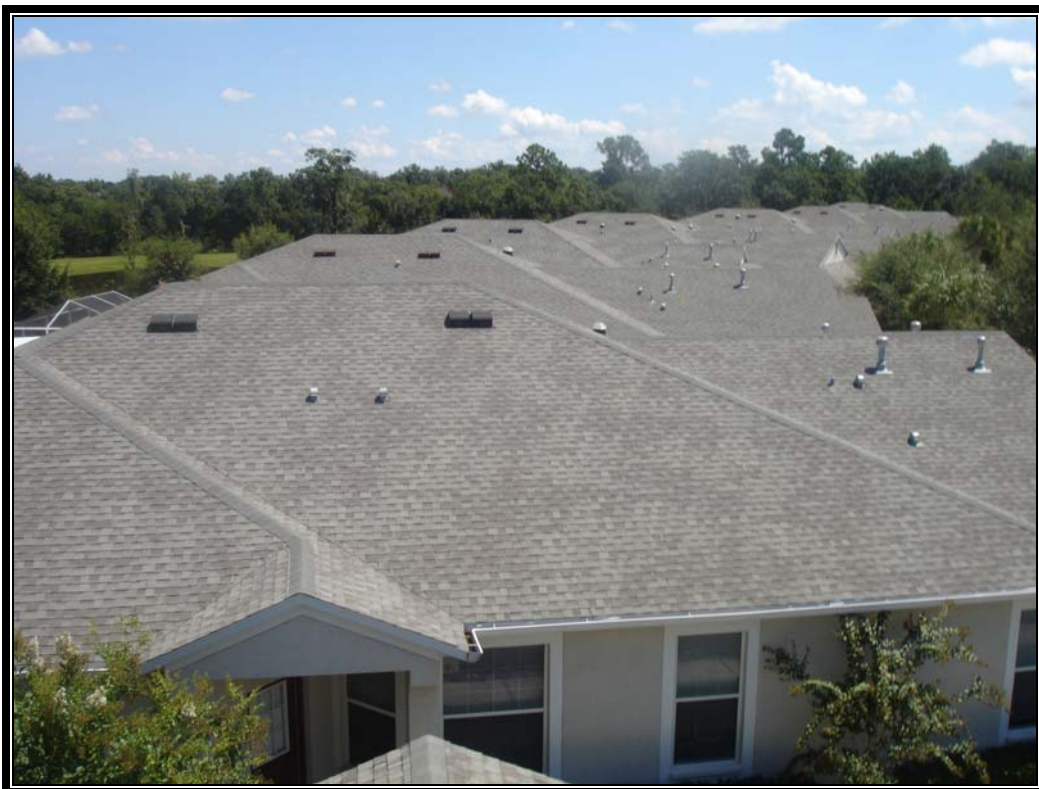
PHOTO #2: ROOF OVERVIEW - TYPICAL
